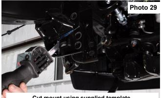
Cut mount using supplied template.
