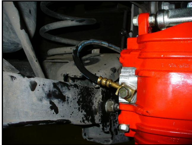
Figure 3: Incorrect installation. Hose installed in this manner will be crushed by the bump stop!!
